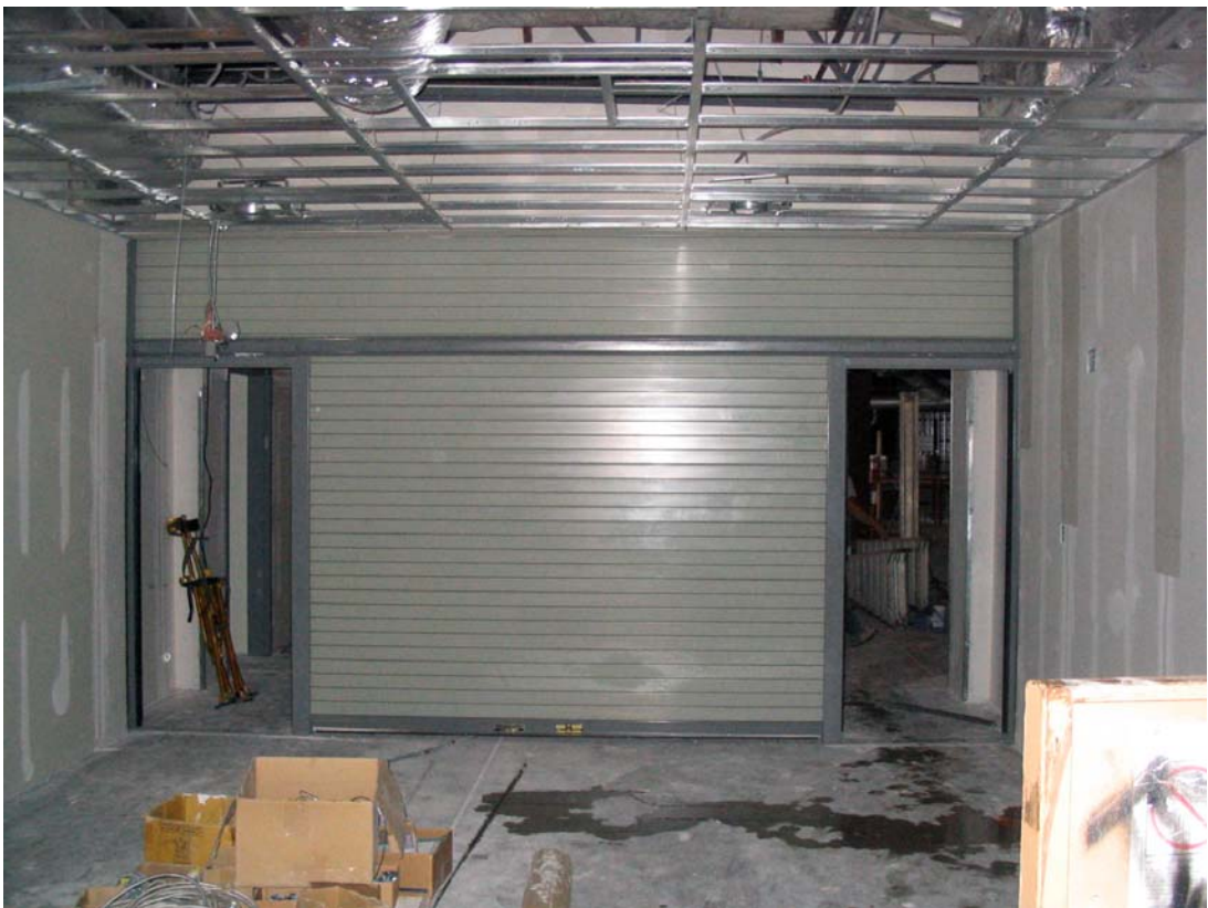
Fire doors and gates being installed
