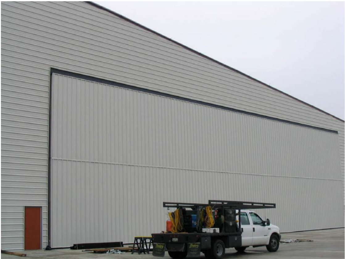
Siding up on exhibit hangar bi-fold door
