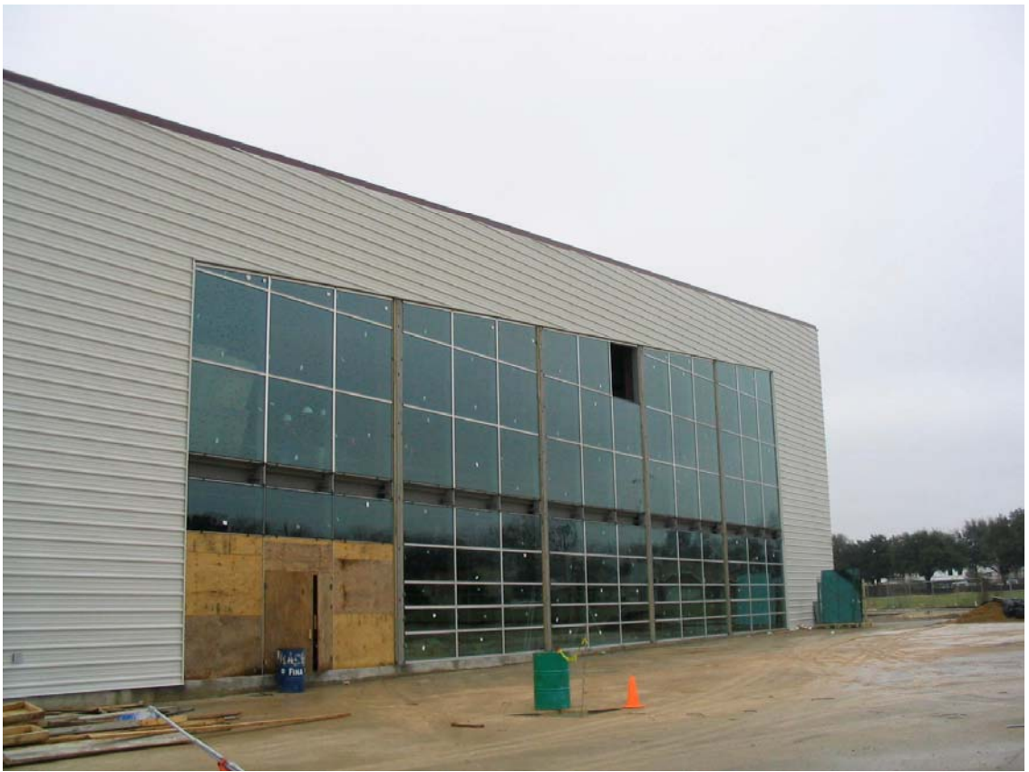
Exhibit hangar windows installed
