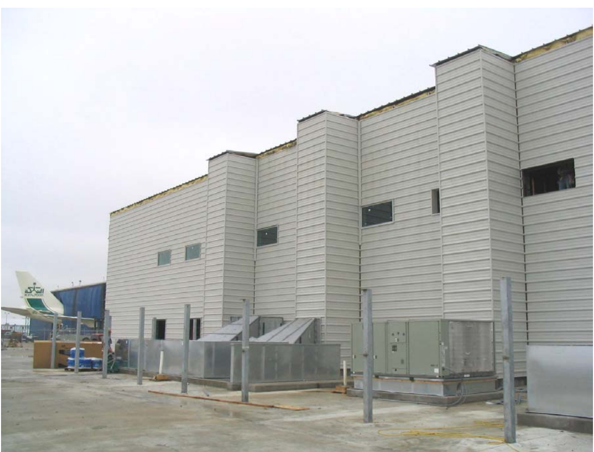
Staff office windows on mezzanine of exhibit hangar
