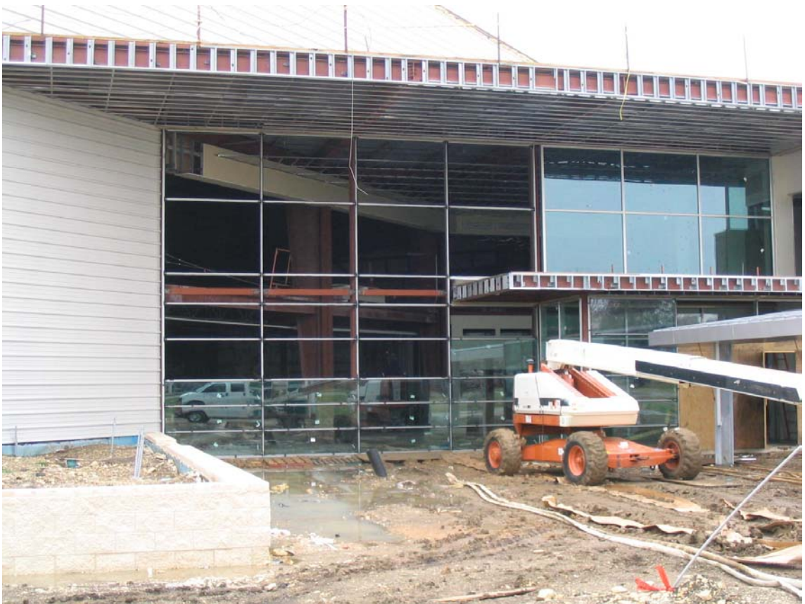
Lobby window frames being installed
