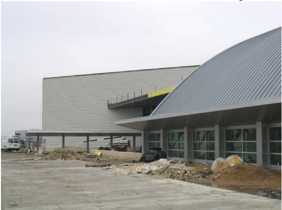
Exterior is taking shape
