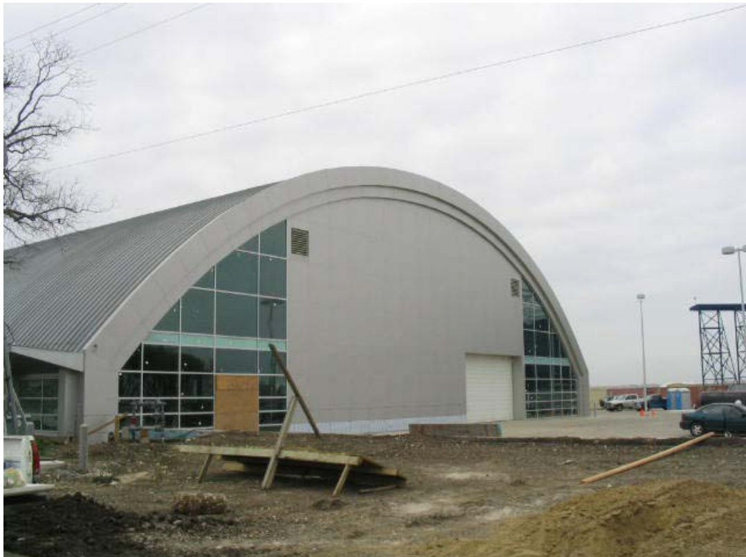
North end of facility
