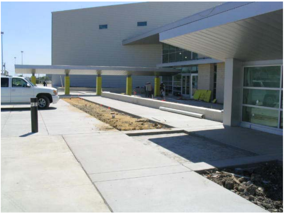
Front entry concrete work completed
