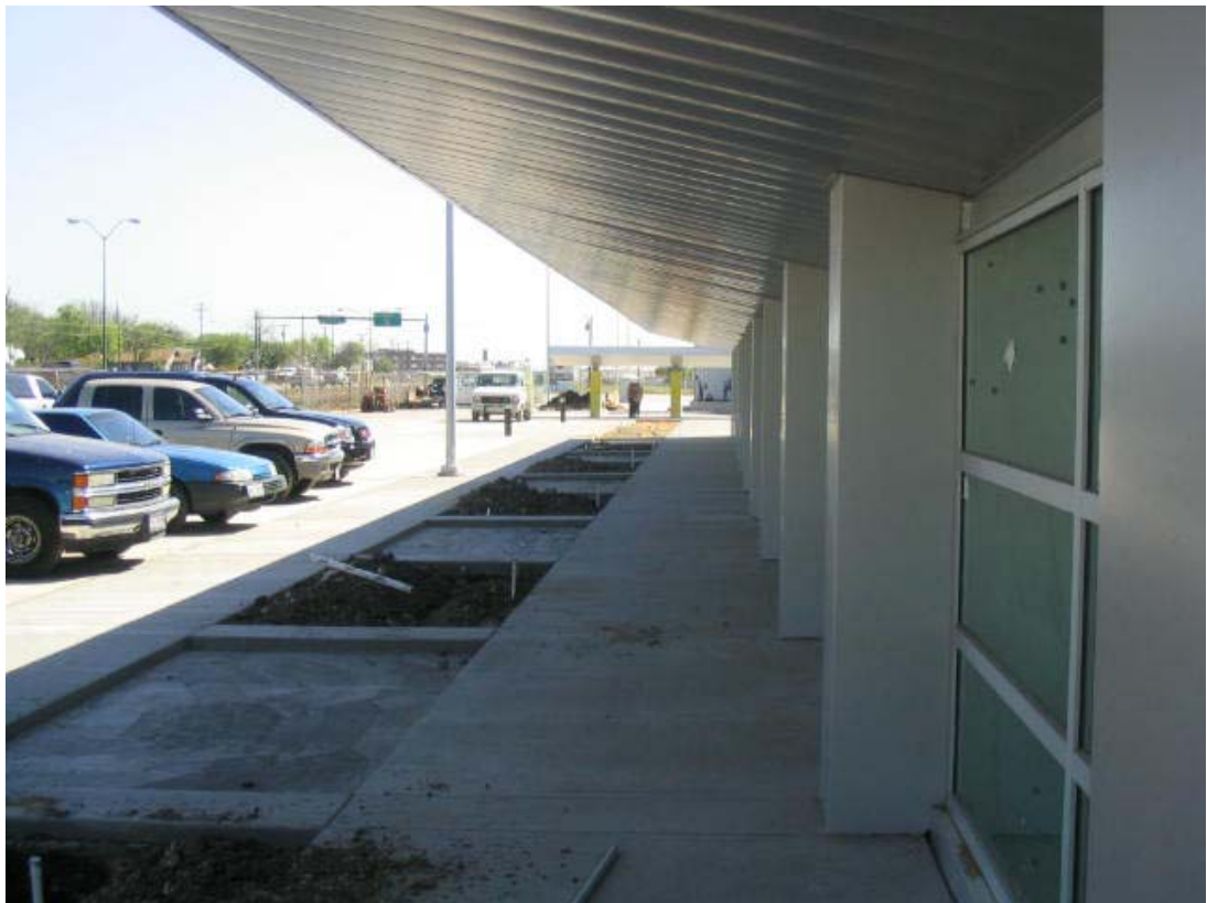
Pavestone bricks and planting areas along front facade
