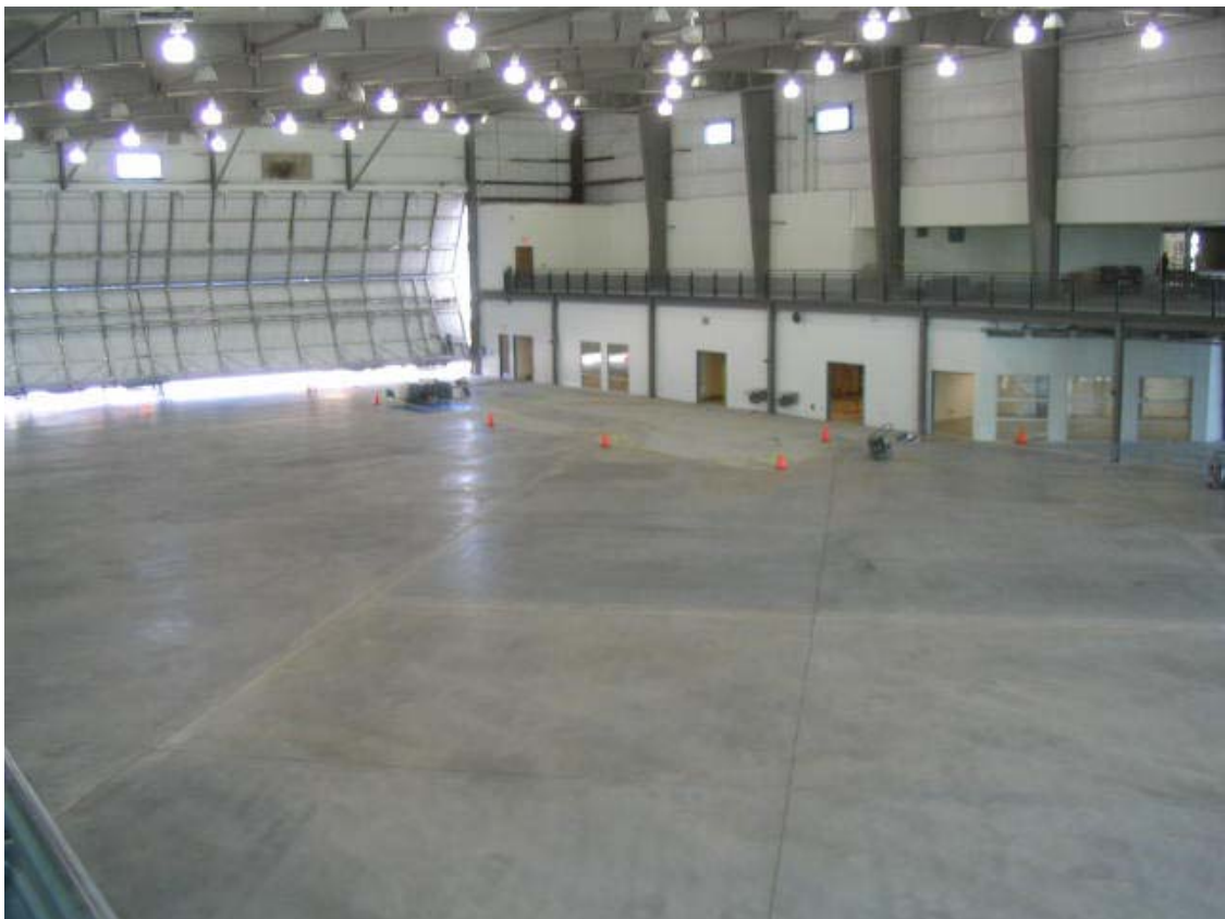
Main hangar deck cleaned and ready for color staining
