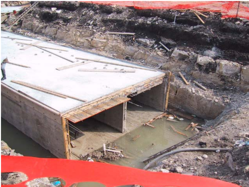
Business end of the culvert
