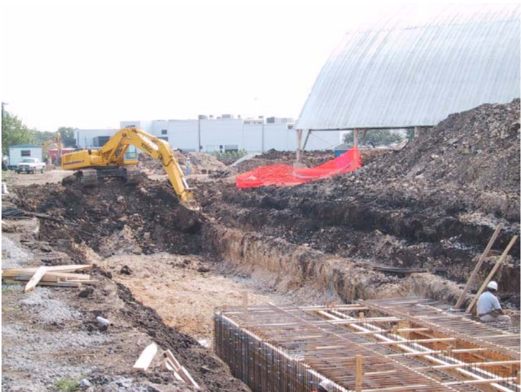
Culvert nearing north end
