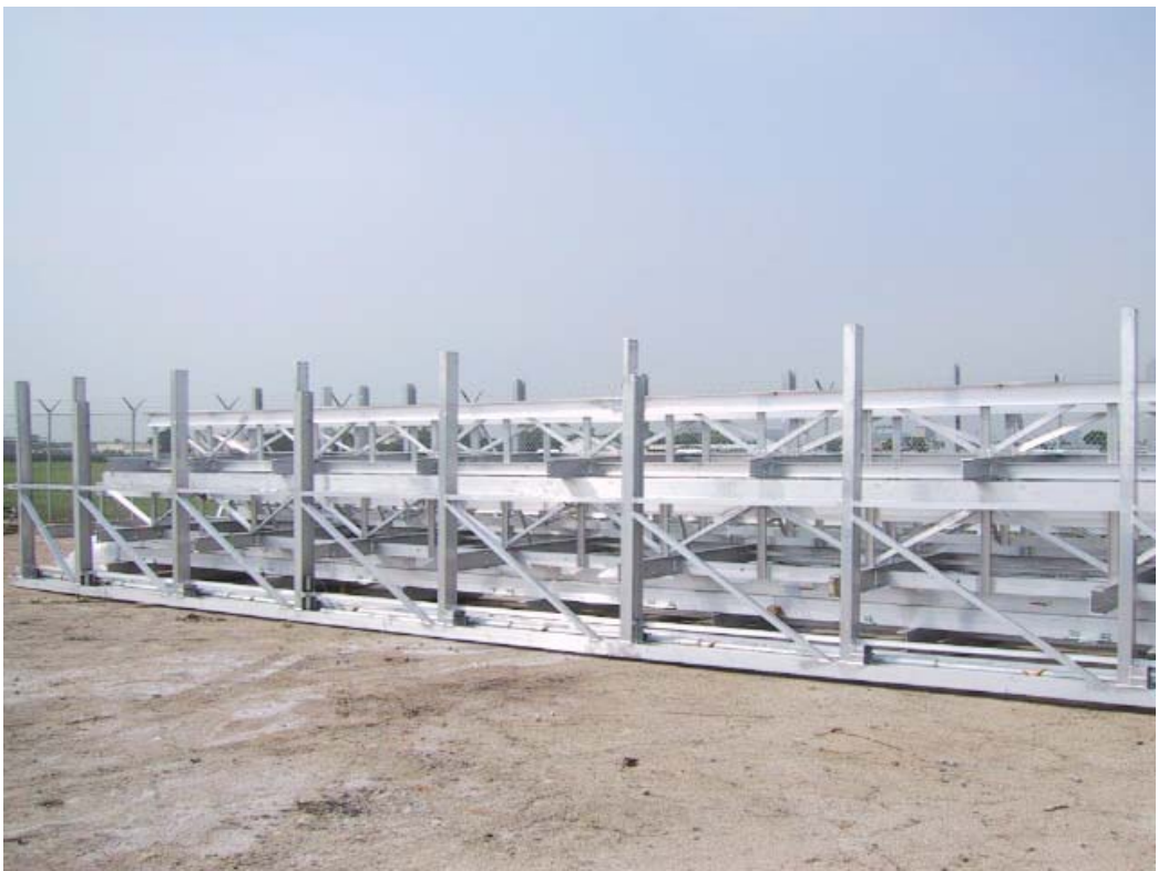
Structure arrives for 110' x 24' main hangar door
