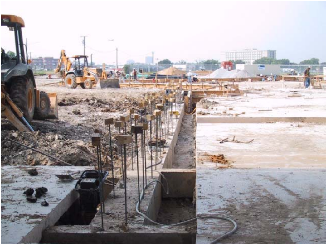
Grade beam being formed
