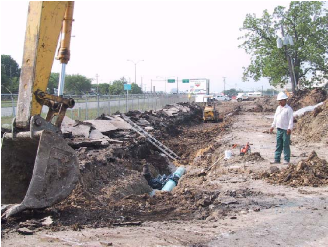
Water main along Lemmon side being completed
