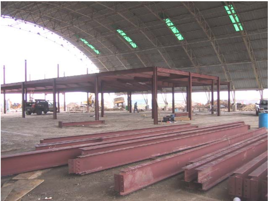
2 nd floor structure for auditorium
