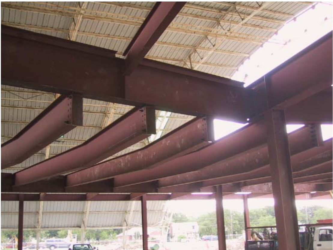
Looking up at auditorium floor beams
