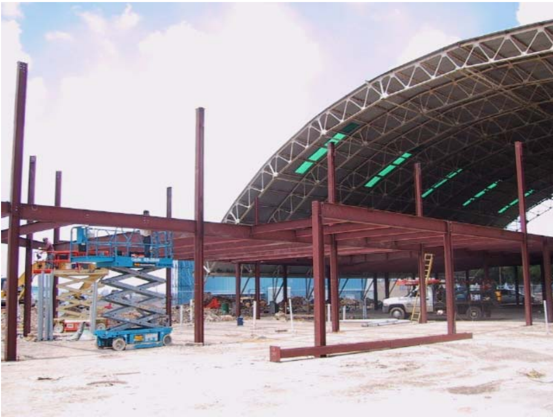
Structure grows from under old hangar
