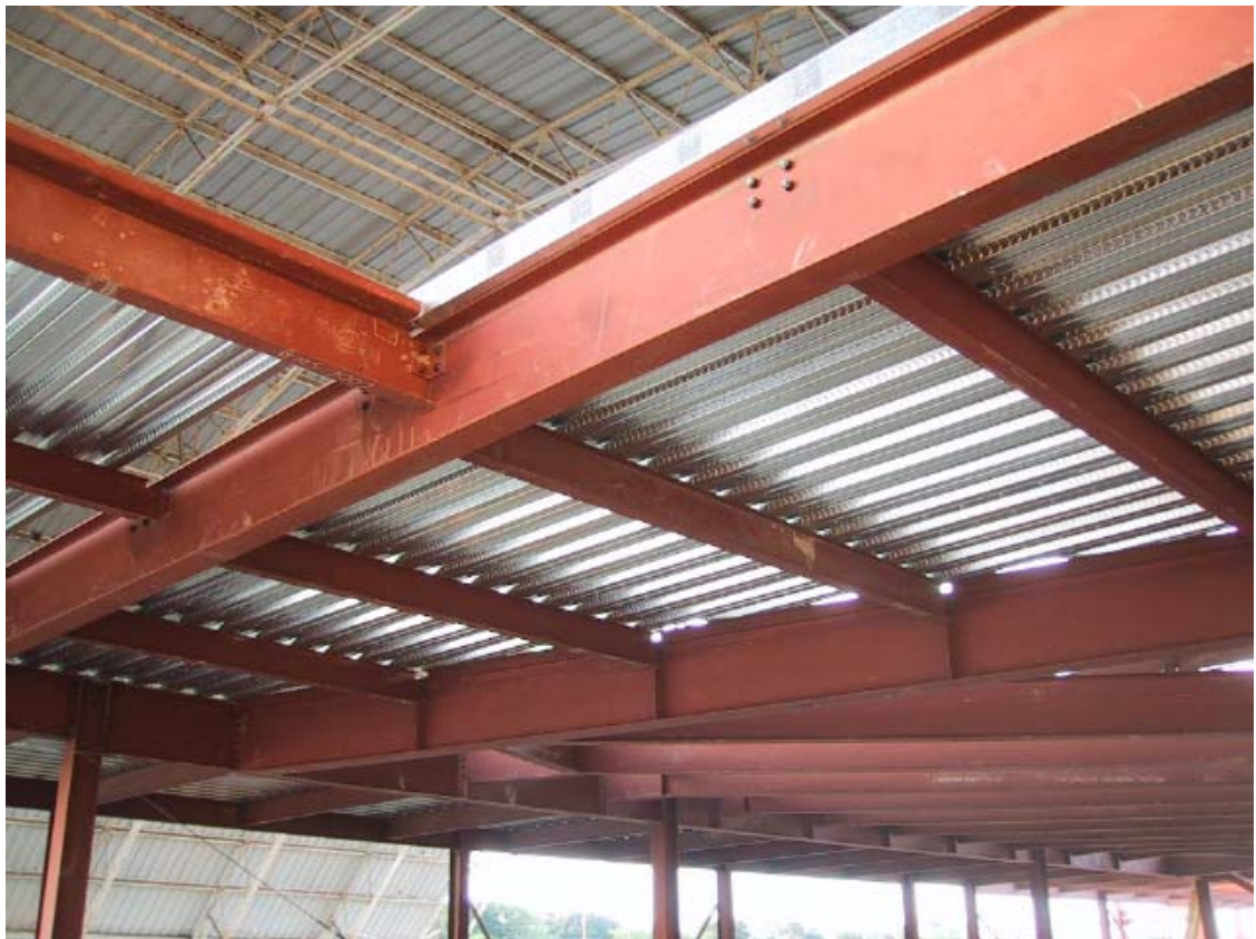
2 nd floor decking being installed
