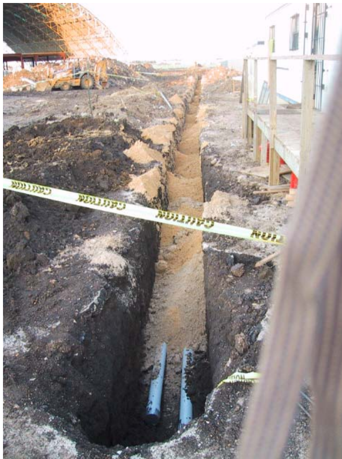
Underground electrical power making its way onto site
