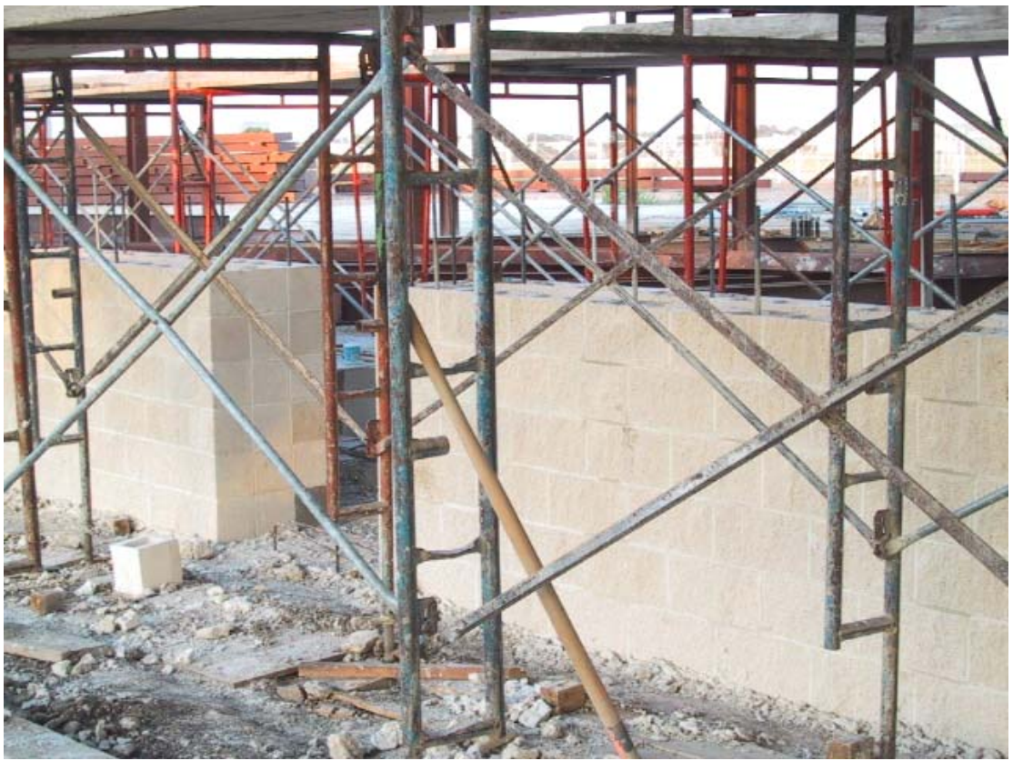
Front façade masonry wall going in
