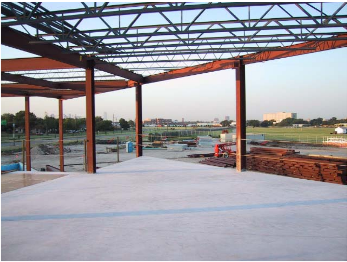
2 nd floor area overlooking main hall floor
