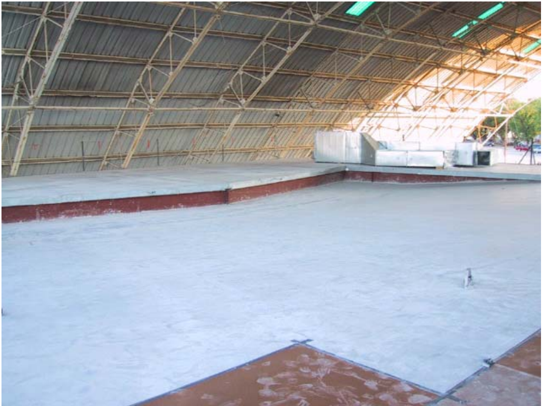
2 nd floor auditorium floor poured
