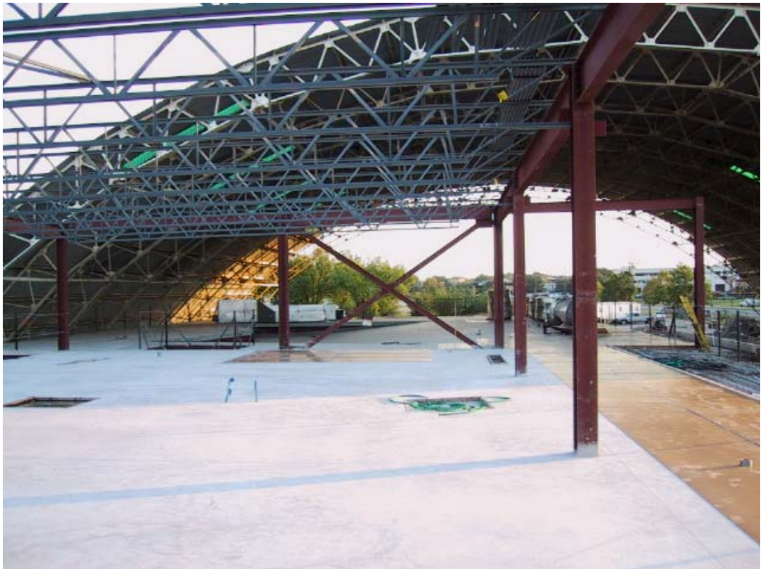
2 nd floor poured looking north
