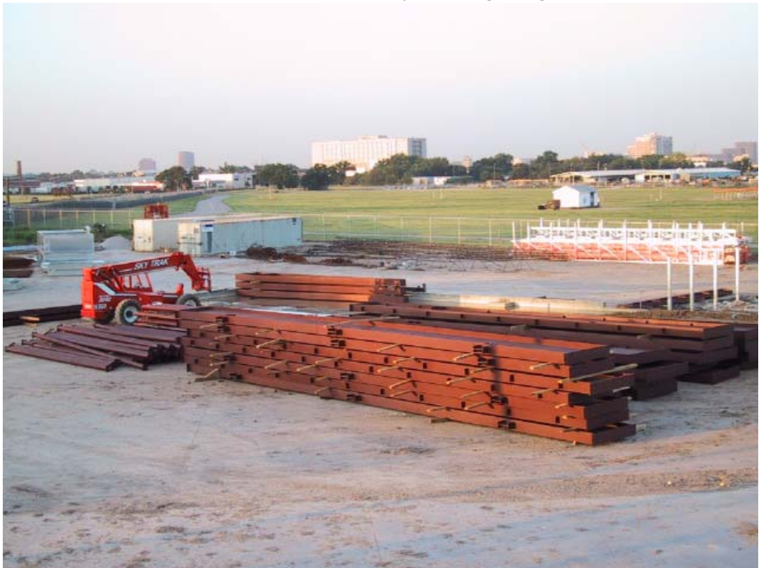
Steel for main exhibit hall has arrived!
