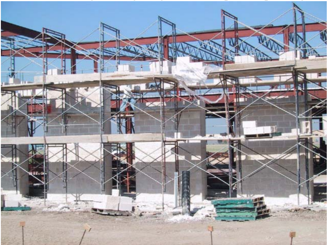
Front façade masonry work continues
