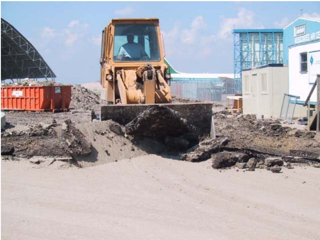
Parking lot work starting
