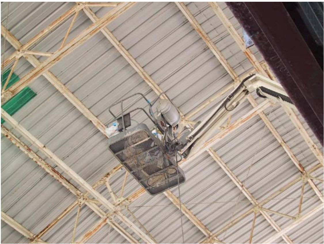
Sandblasting existing hangar structure prior to painting
