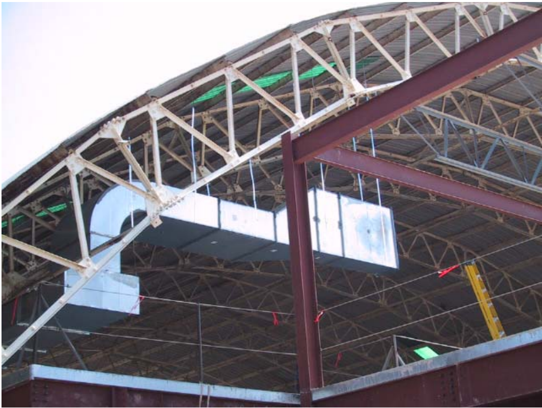
HVAC duct work starting to go in
