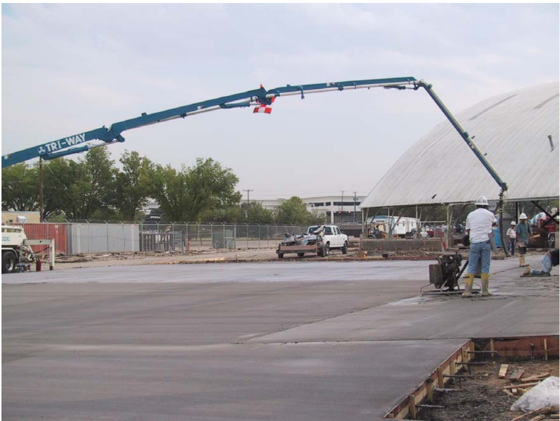
Pouring north end portions of parking lot
