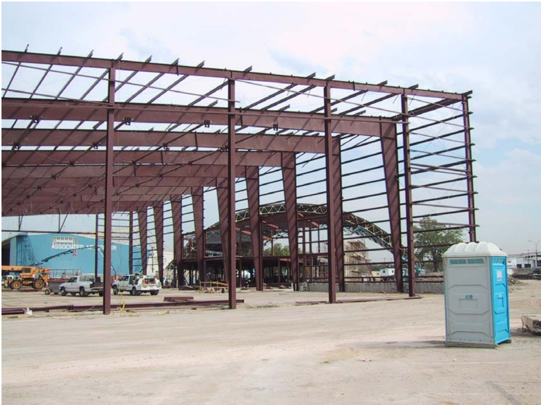
Outside structural steel for new hangar nearly complete
