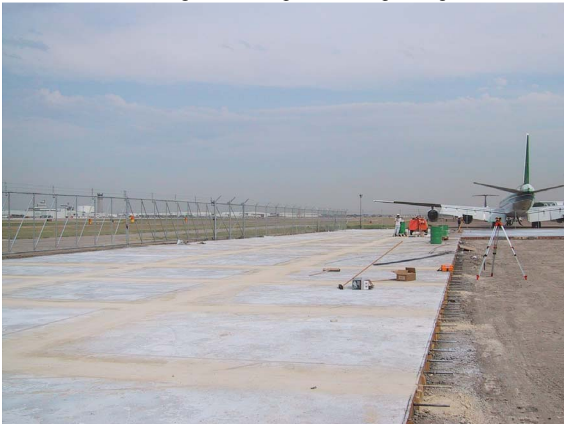
Poured parking lot along west fence line
