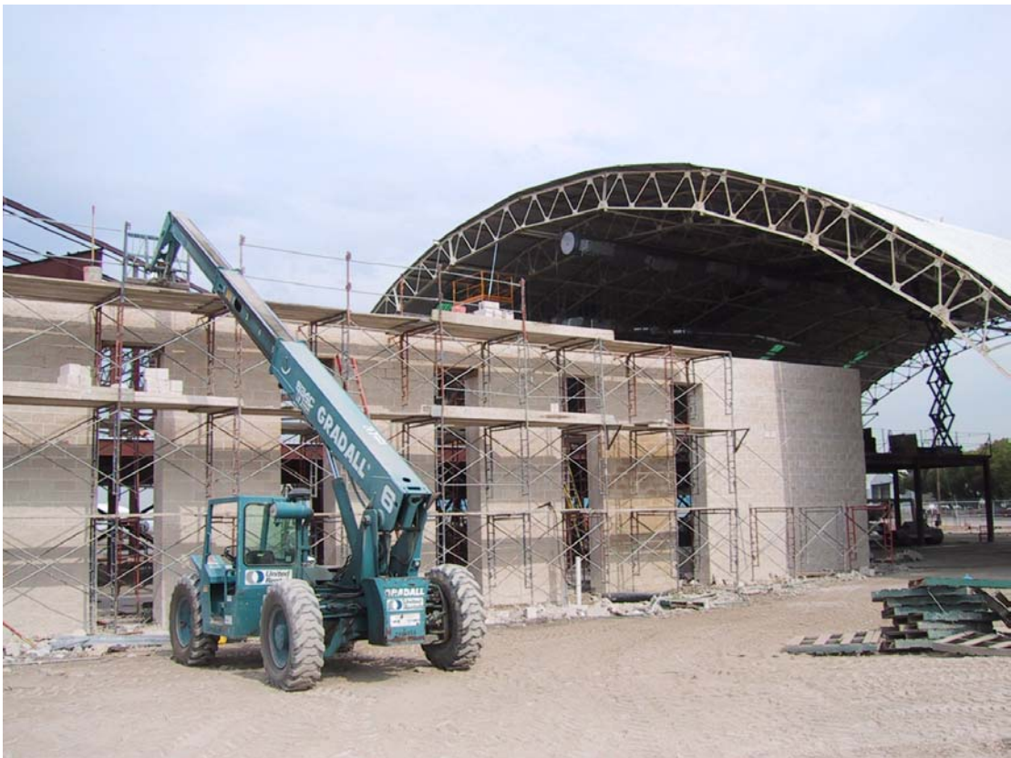
Topping out of masonry wall
