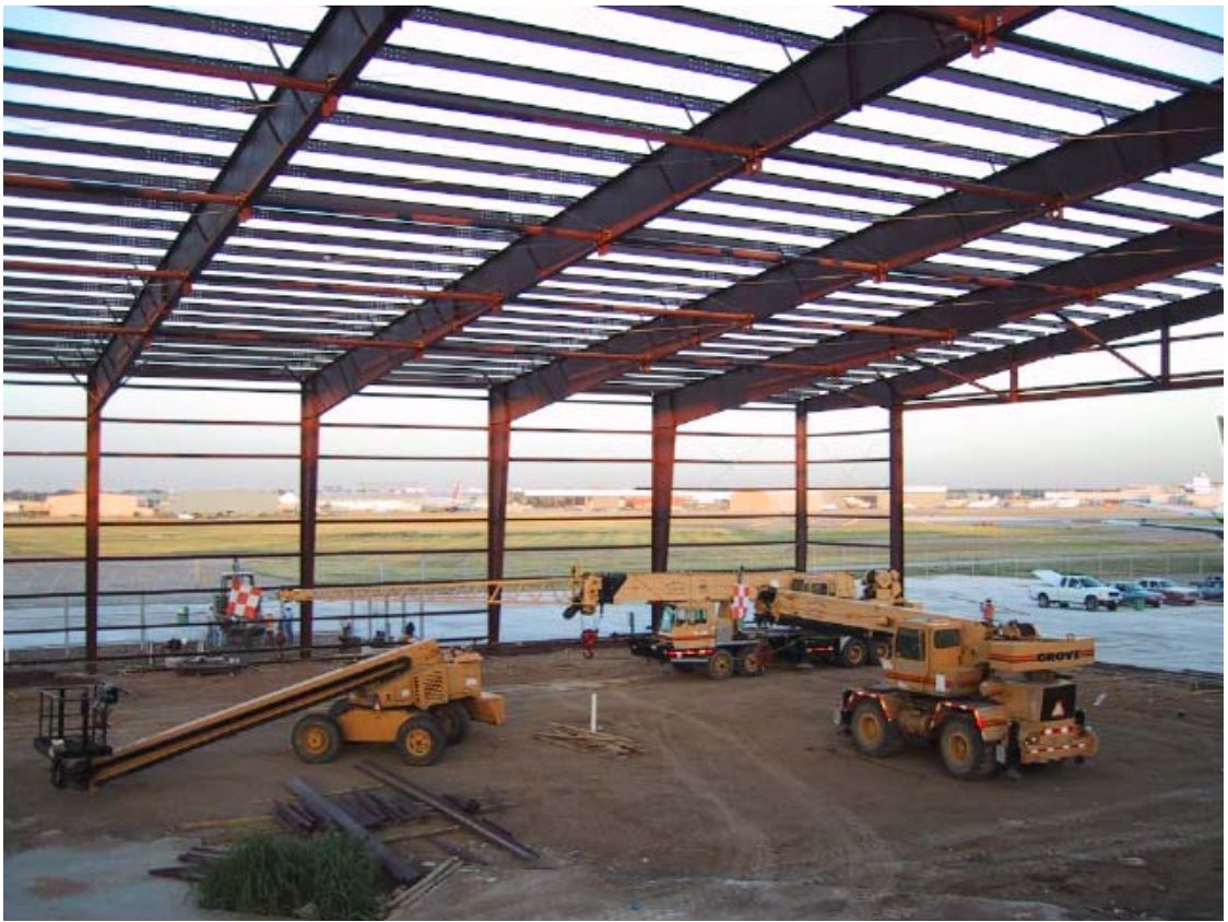
View towards runway
