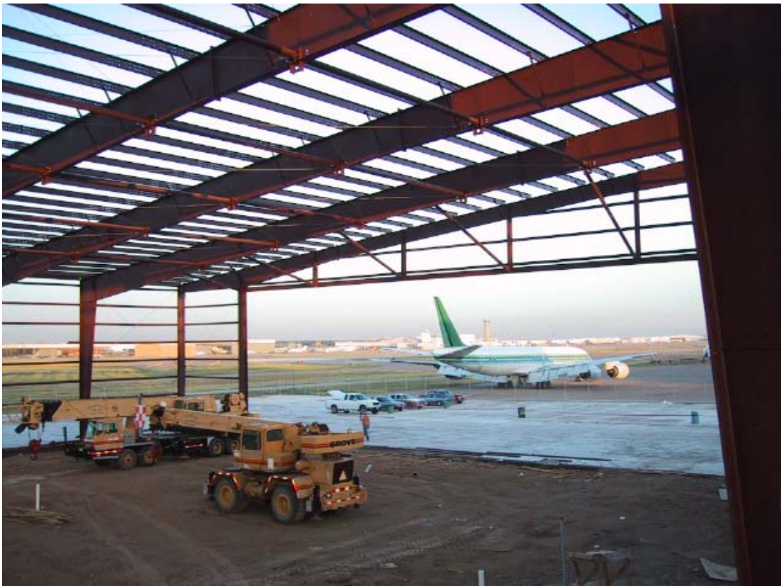
View north out of new exhibit hall
