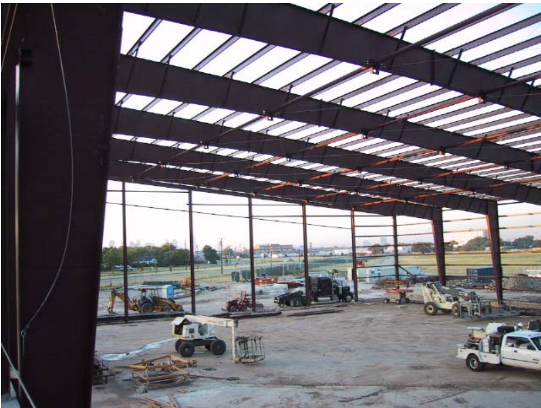
View towards Lemmon from inside new exhibit hall
