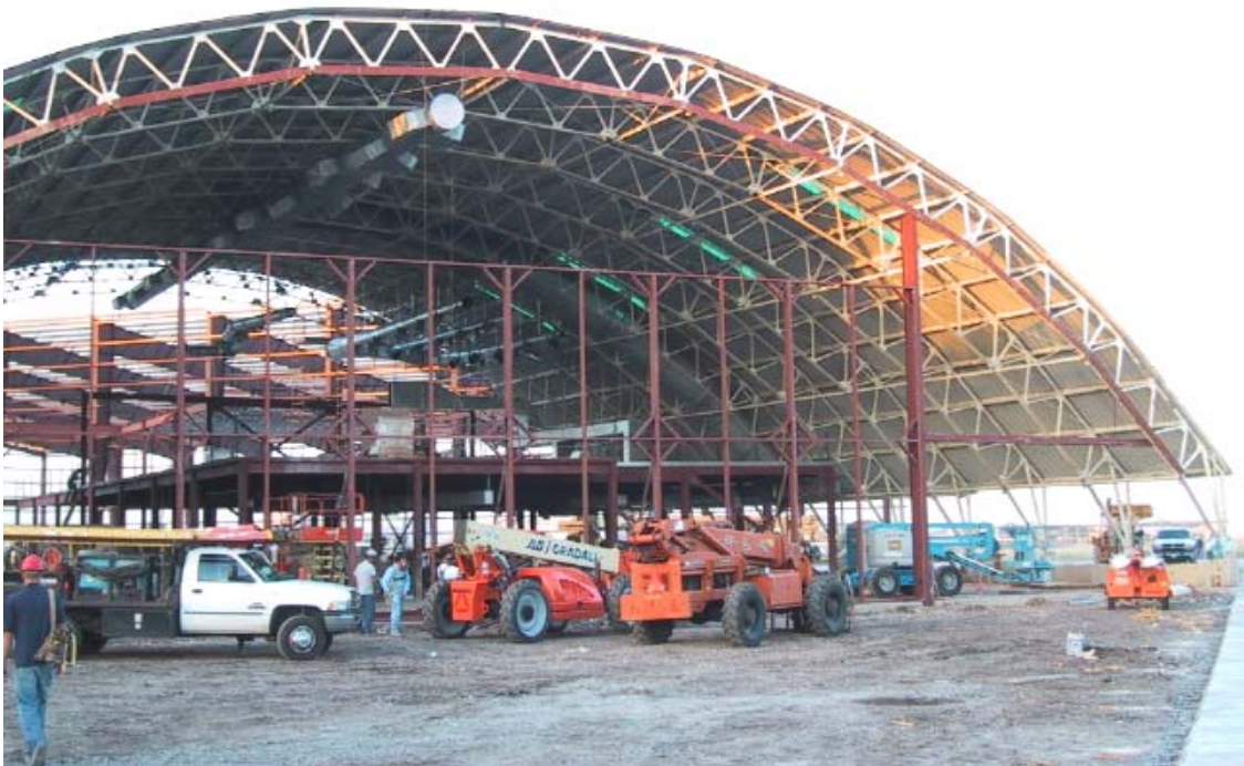
North end of existing hangar going up
