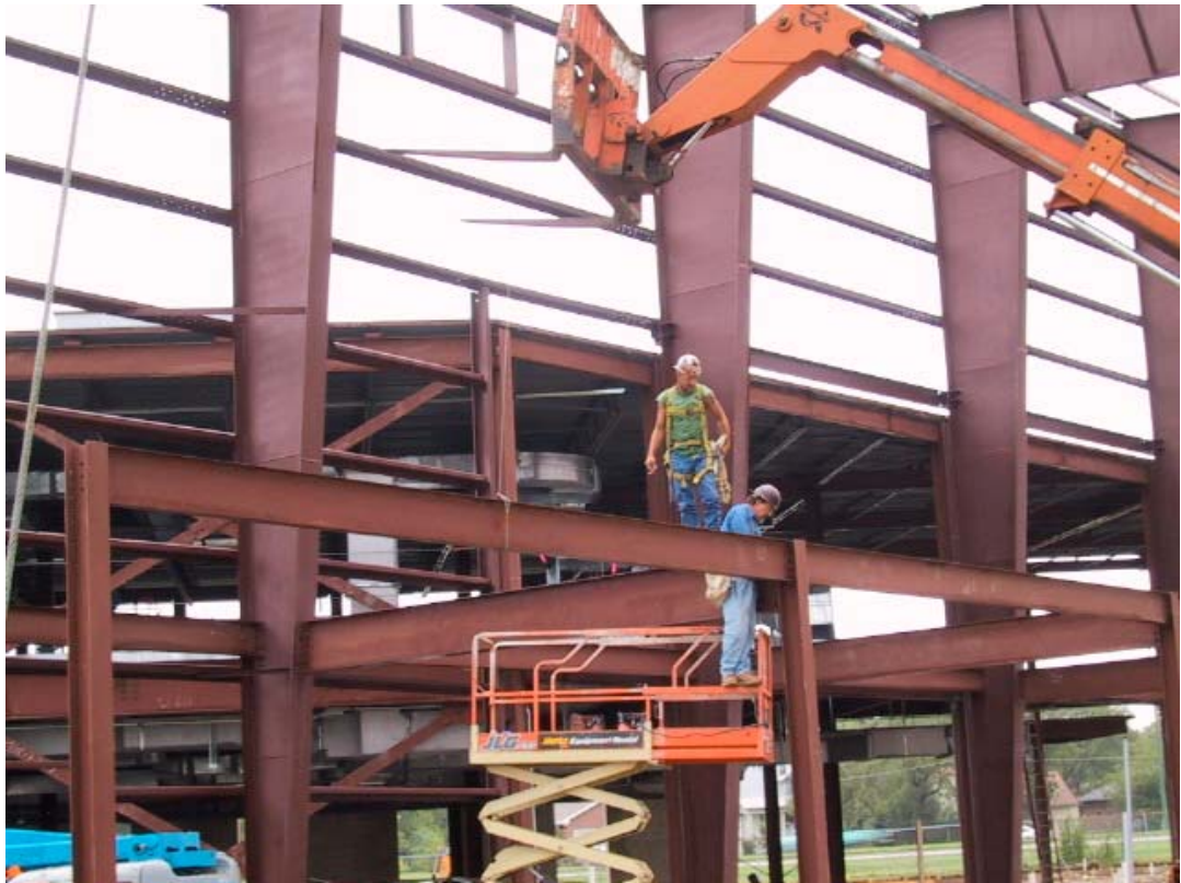
2nd floor mezzanine going up in main hall - shot 2
