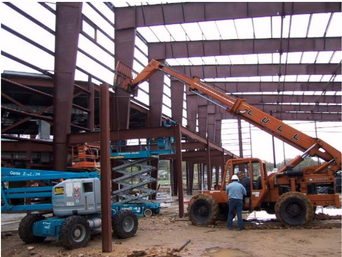
2nd floor mezzanine going up in main hall - shot 1
