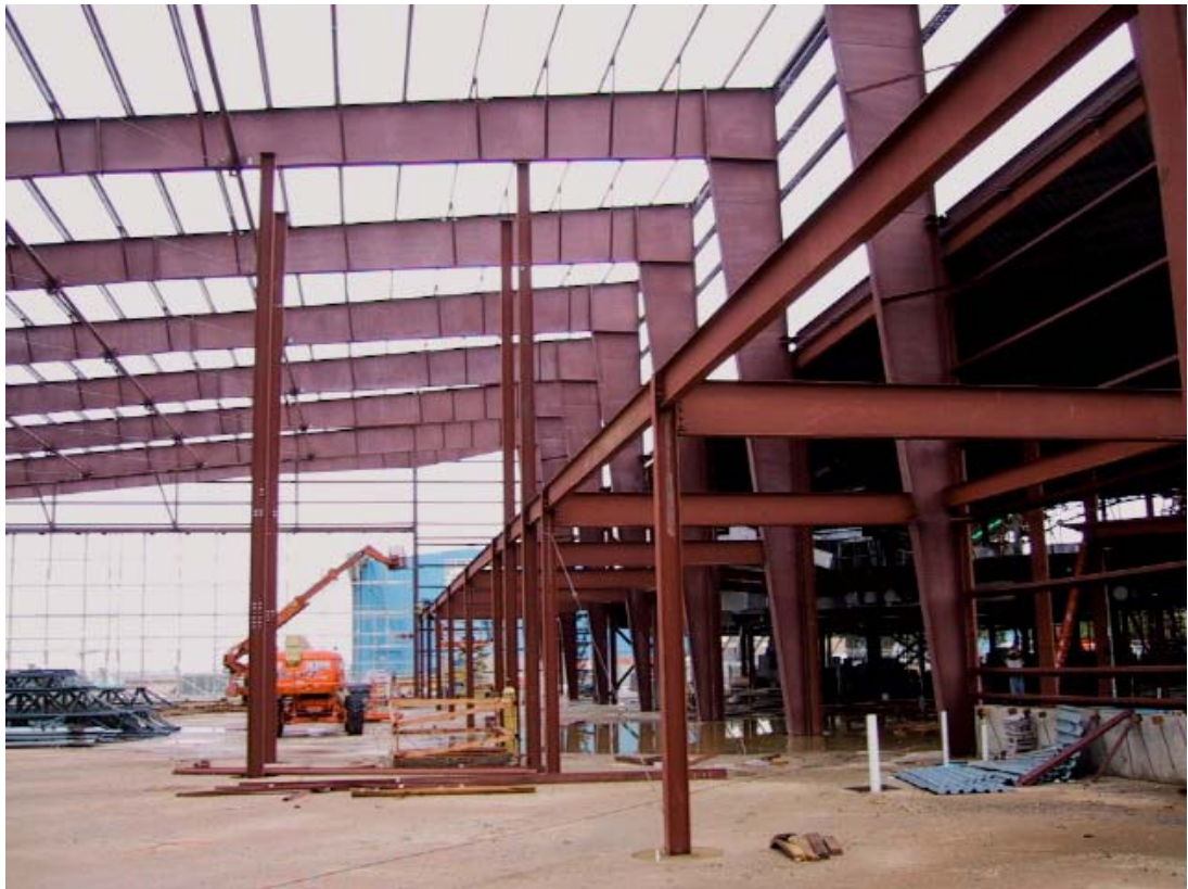
Mezzanine columns-east side (Note elevator tower columns)
