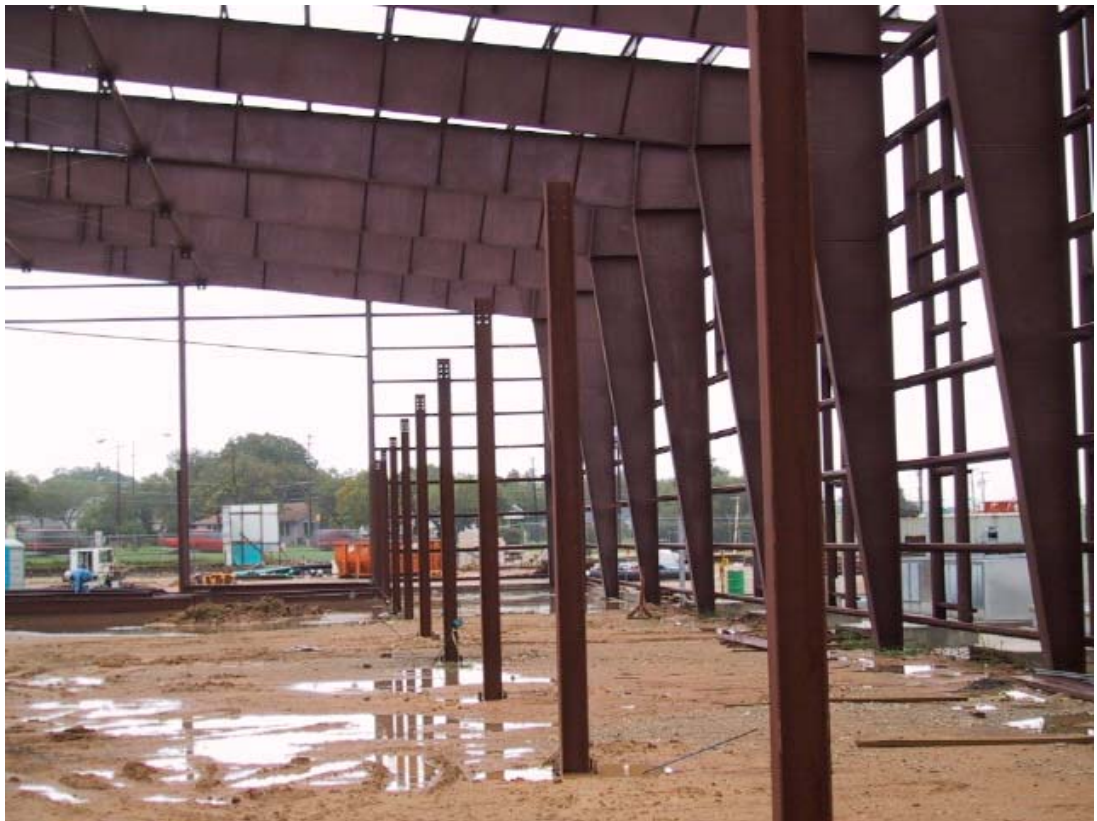
Mezzanine columns-west side
