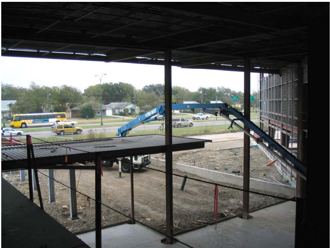
Concrete pumper
