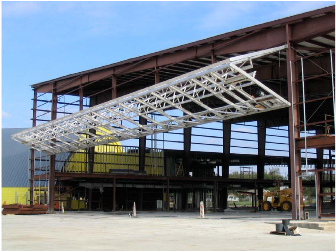
Exterior view of hangar door
