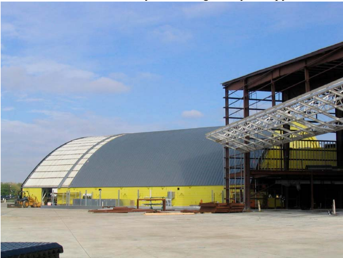
Last few roof panels going up on backside of old hangar
