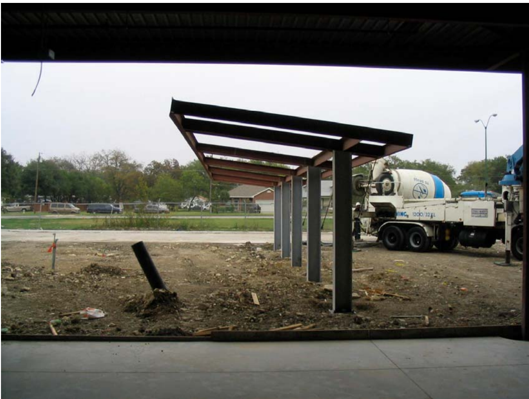
View from lobby out through entry canopy
