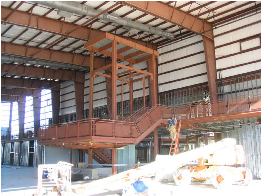
Railing install continues around elevator and stair landing
