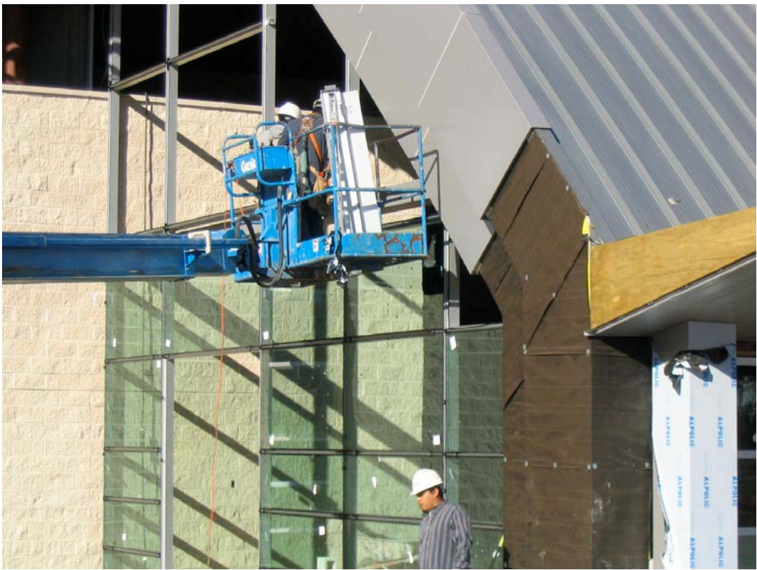
Glass being installed on south end of renovated hangar
