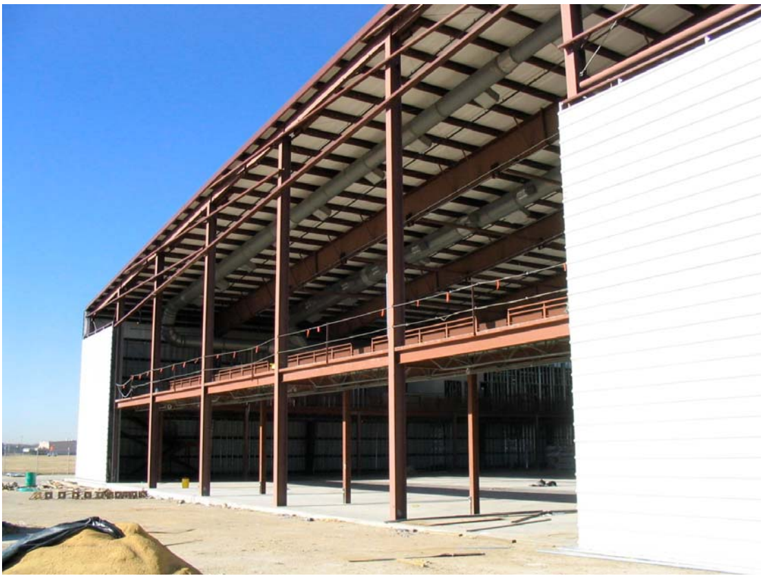
South end siding and window area of main hangar
