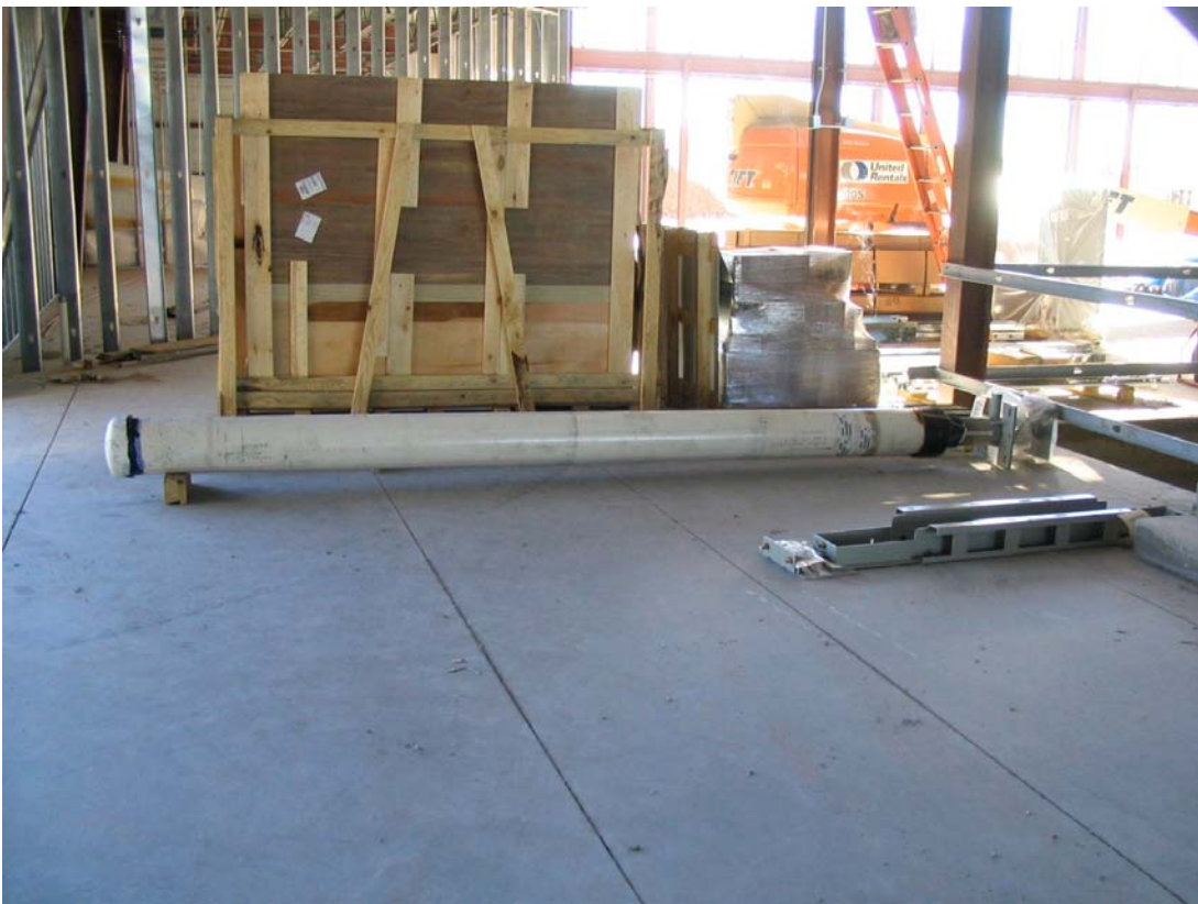
Visitor elevator equipment has arrived
