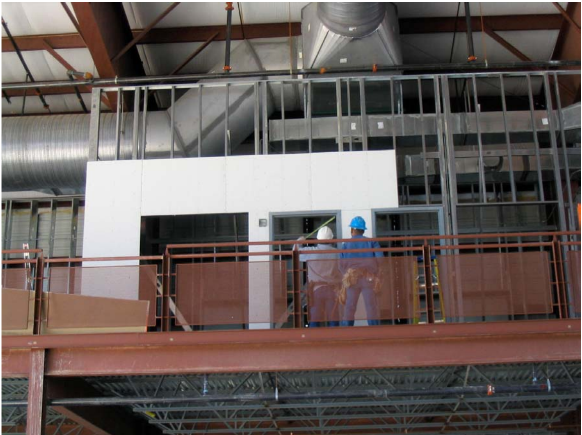
Staff offices being sheetrocked
